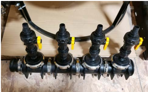
Dura Auto-Batch™ Direct Injection 3" Kit Assembly
